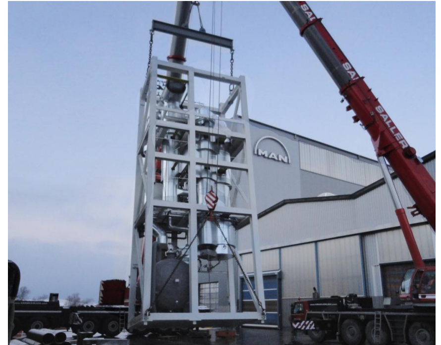
MES methanation reactor for the Power-to-Methane plant in Werlte (world's largest methanation plant)
